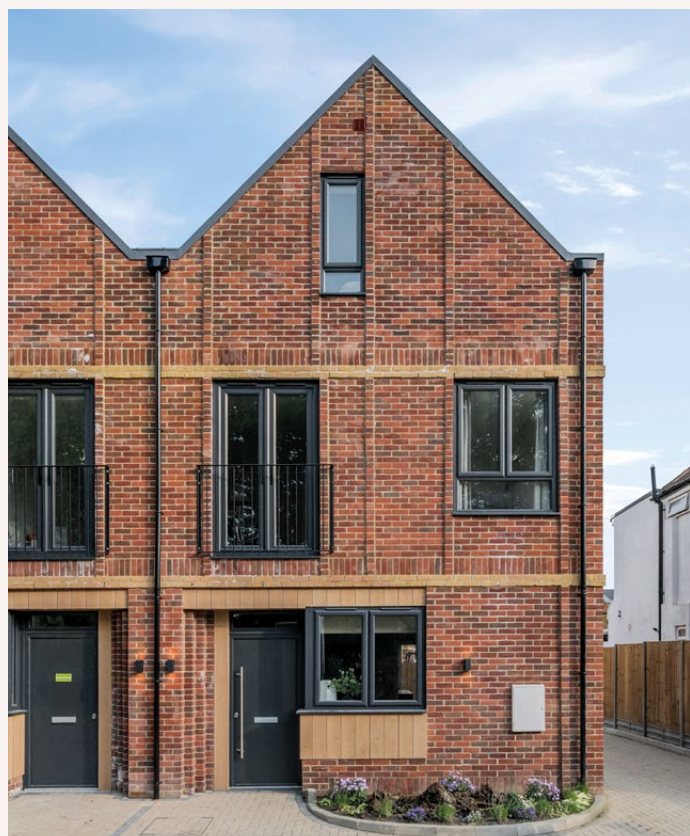
Bramley Road, Oakwood, N14 4HA Scarlet Oaks, developed by Amara Property.
